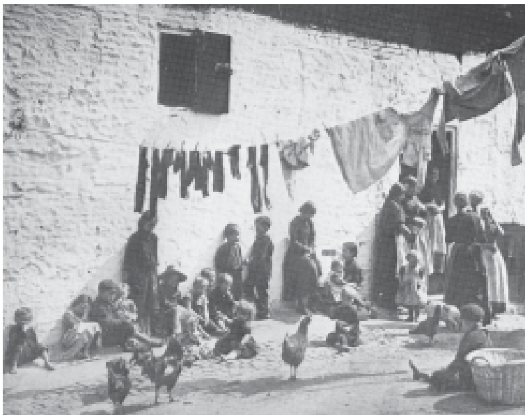
Fig. 4 – A London slum in 1889. What are the different uses of street space that are visible in this picture? What would have changed in the conditions of working class housing in the twentieth century?
