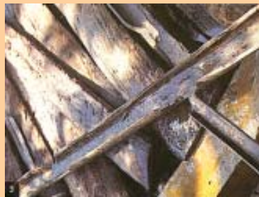
Picture 2 and 3: The channel sections, made of bamboo, divert water to the plant site where it is distributed into branches, again made and laid out with different forms of bamboo pipes. The flow of water into the pipes is controlled by manipulating the pipe positions.
