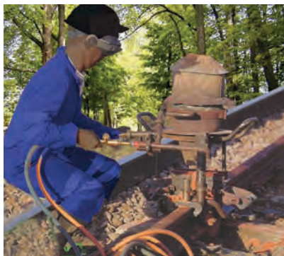
Figure 3.11 Thermit process for joining railway tracks
